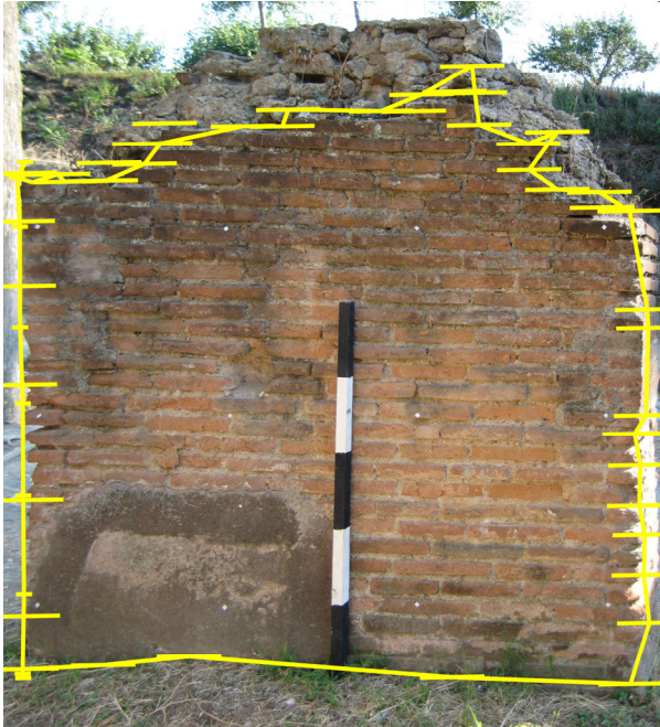
Figure 9. Comparison of Type One result with surveyed surface outline.
