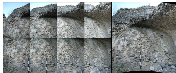
Figure 7. Original images and stitched rectified result of a wall surface using Type Two method.
