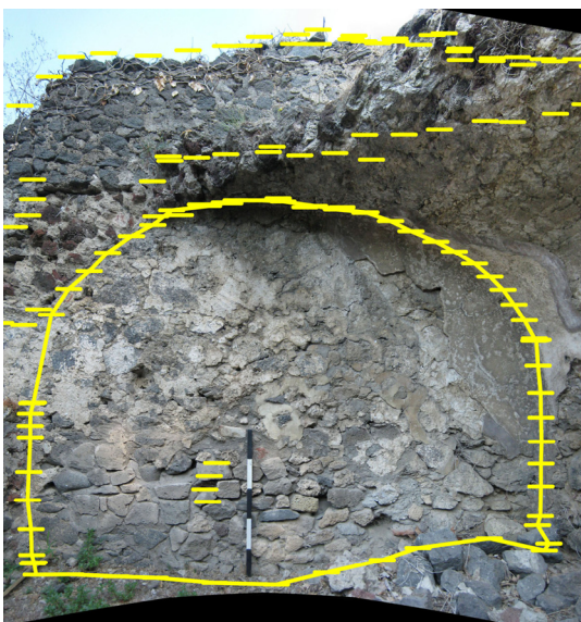
Figure 10. Comparison of Type Two result with surveyed surface outline.
