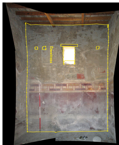
Figure 13. Comparison of rectified wall surface with surveyed wall outline demonstrating use for stitching well-preserved wall painting.
