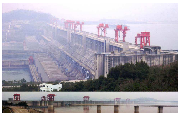
Figure 19 The Three Gorges Dam in 2008 (above) and the sediment-choked, impounded Yangtze River right upstream the dam in 2010 (below). Pictures were taken by S. Schönbrodt-Stitt.
