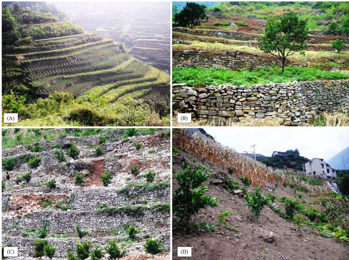
Figure 7 Examples of the different terrace condition classes from the backwater area of the Xiangxi catchment; (A) ‘well maintained’ (A), ‘fairly maintained’ (B), ‘partially collapsed’ (C), and ‘completely collapsed’ (D). Photos by S. Schönbrodt-Stitt.
