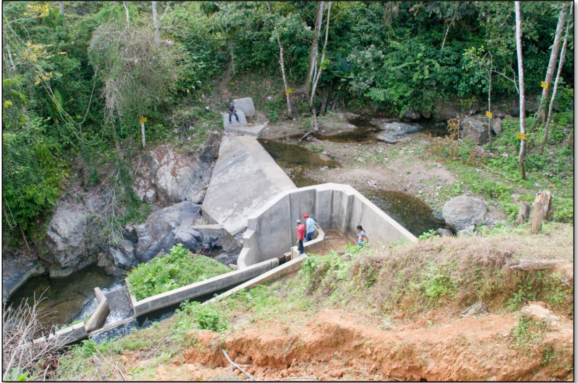
Water intake for PCH El Naranjo
