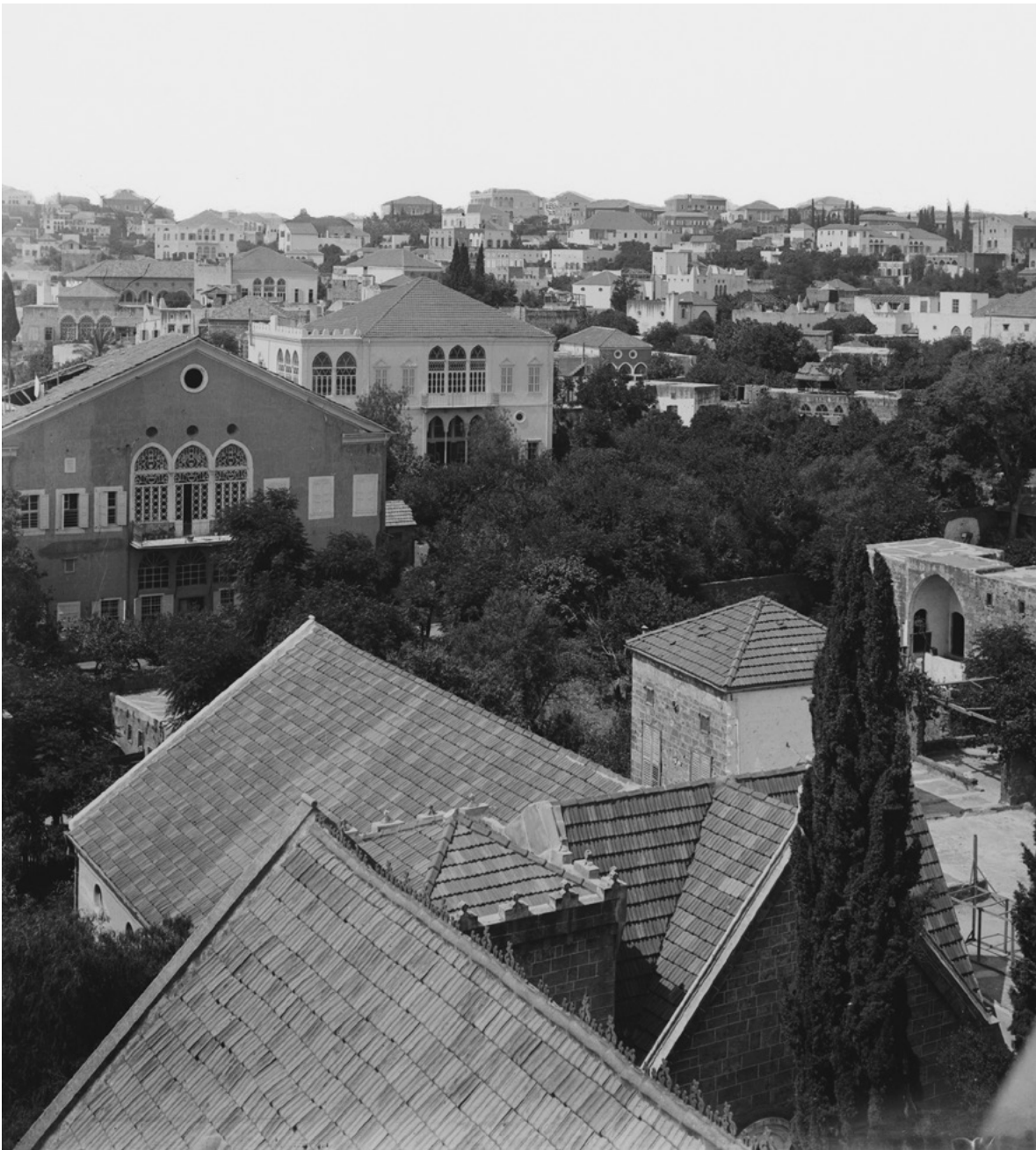
Figure 1: A View of Central Hall Houses in Beirut with Tiled Roofs, Triple-arch Windows and Balconies. Source: Matson (G. Eric and Edith) Photograph Collection, Prints and Photographs Division, Library of Congress Online Catalog, Call Number LC-M32- 450 [P&P], 1900-1920. https://www.loc.gov/resource/matpc.01183 (accessed 14 September 2020).
