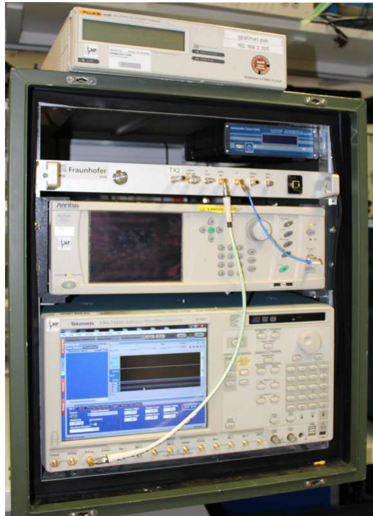
Figure 6.8: The transmitter unit for the bistatic radar measurements developed by Fraunhofer FHR. On top of the green box the Rubidium standard is located, providing the external generated 10 MHz signal.
