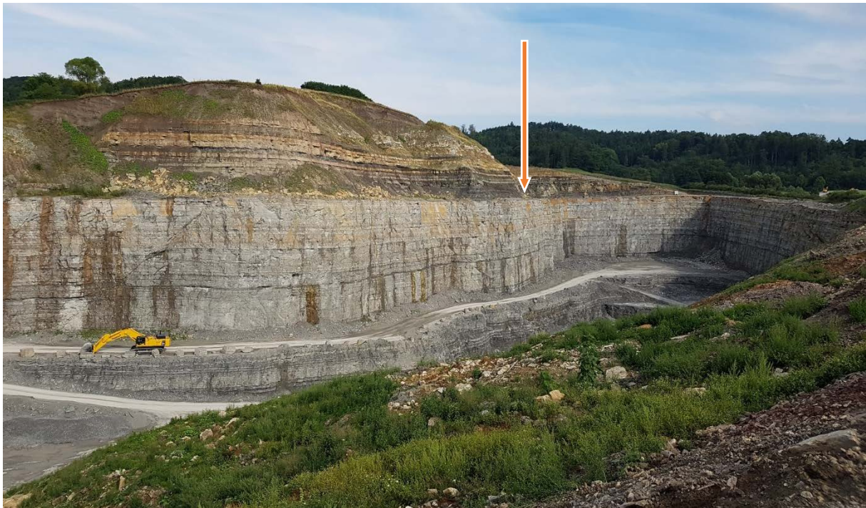
Figure 6: Panoramic view of Schumann quarry. The massive grey banks are Muschelkalk layers, the yellowish and dark grey sediments lying atop are Keuper sediments. The arrow marks the excavation site of 2017.
