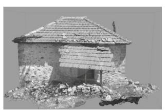
**Figure 5.** Reconstructed model of Building 12 from Aigition, created using iPad videos.
