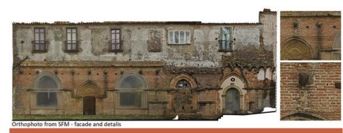
**Figure 9.** Orthophoto of the façade obtained through three different methodologies: High Resolution camera, Structure from Motion and Image Matching, Laser scanning-RGB mode. Comparison about RGB data
