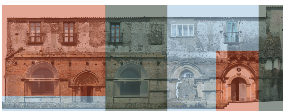
Orthophoto from high resolution camera. Acquisition parameters: ■ 10m, 50mm ■ 5m, 50mm ■ various distances, 35mm
